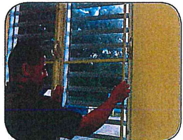
Install or repair window & door screens.
