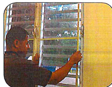
Install or repair window & door screens.
