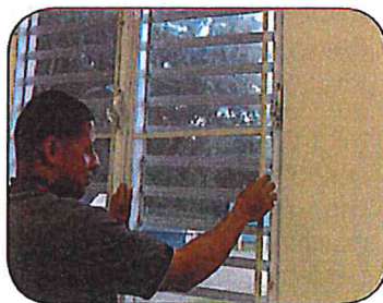
Install or repair window & door screens.
